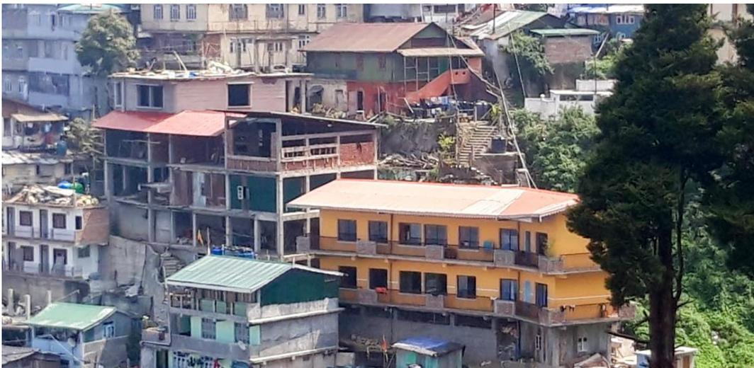
This amazing photo shows the site with the boys' dormitories on the right and the unfinished state of Phase 2. The incomplete brickwork identifies the floor where girls' new dormitories are located. Part of the floor below with its green shuttering is being used as a temporary kitchen. The unfinished staff accommodation is below that. In the background you can see the steps leading to the old
